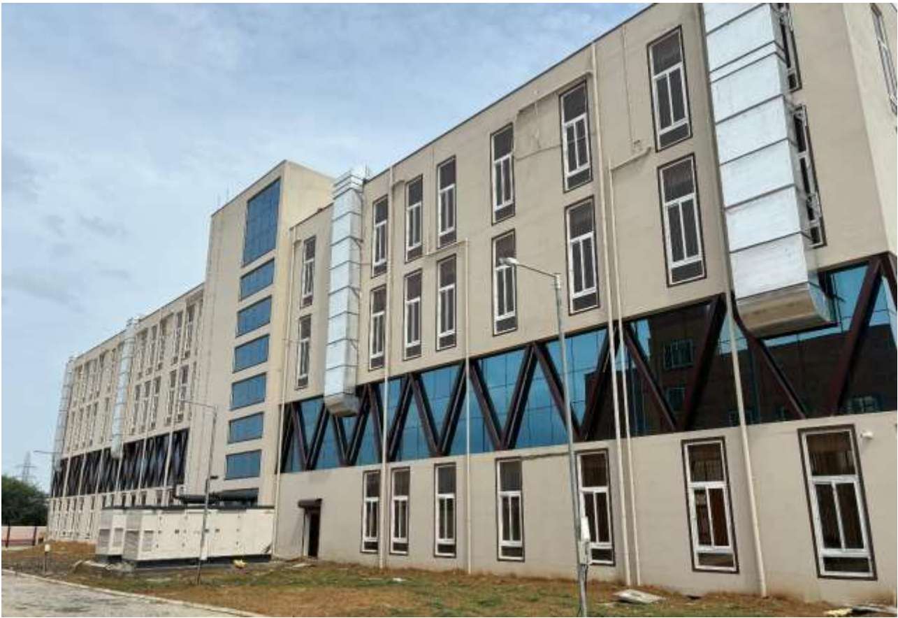
Figure 3.2: Medical Device Park CIF Building in Tamil Nadu
