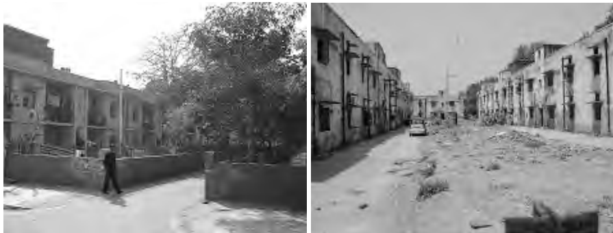
Figure 6: Government Employee Housing Before Redevelopment.
