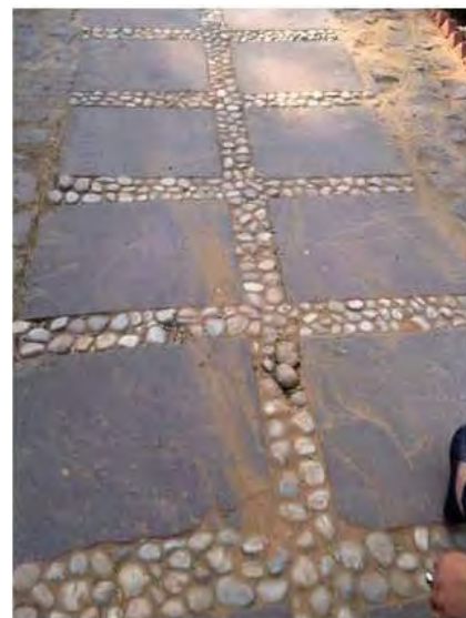
Fig. 9: Pebbles used in pathways to retain rainwater
