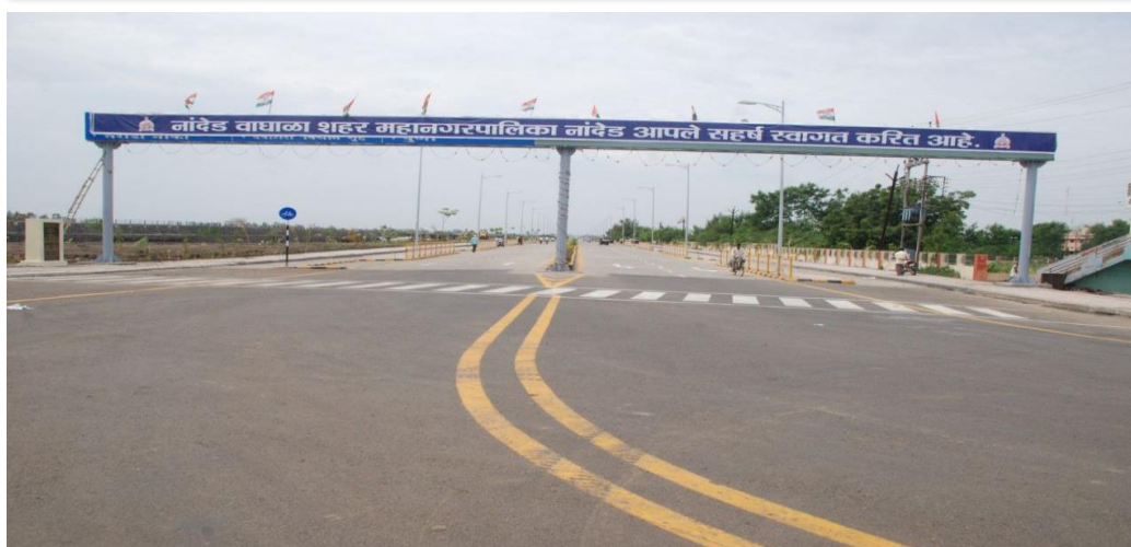
Multiple Lane Roads in Nanded
