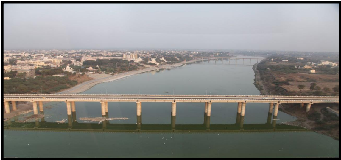
Bridge on Godavari river
